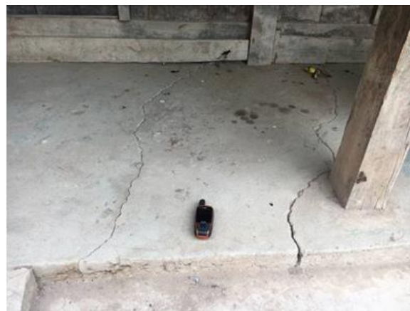
Figure 4. Cracks appeared inside the office of the People's Committee (left) (L2 in Figure 3) and in a nearby house (right).
