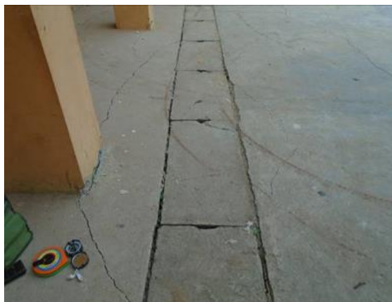
Figure 4. Cracks appeared inside the office of the People's Committee (left) (L2 in Figure 3) and in a nearby house (right).
